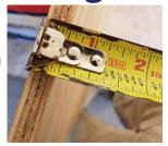
6 photos showing roof deck nailed down with 8d ring shank nails with the max. distance between nails being 6" and nails marked with marker or chalk
